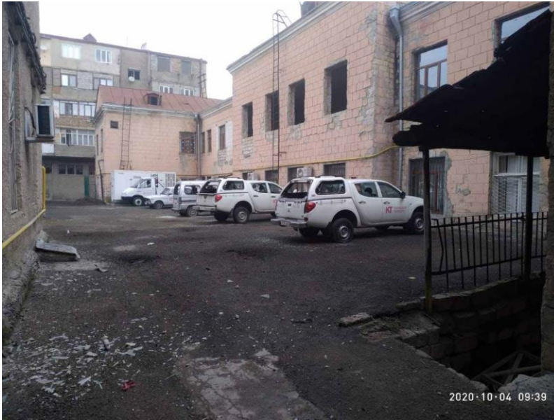
Figure 59. The Head Office of the Telecommunication Company Struck by Azerbaijan
