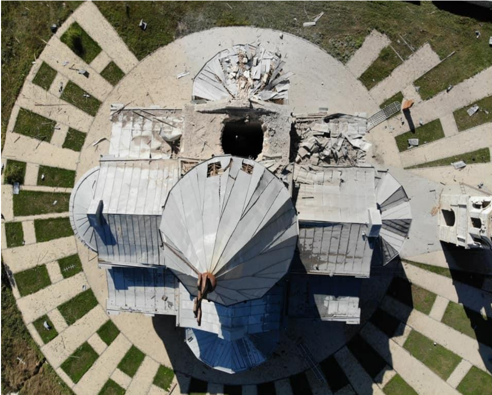
Images 1-4: The damage caused to the Holy Savior Ghazanchetsots Cathedral following the two strikes on 8 October 2020
