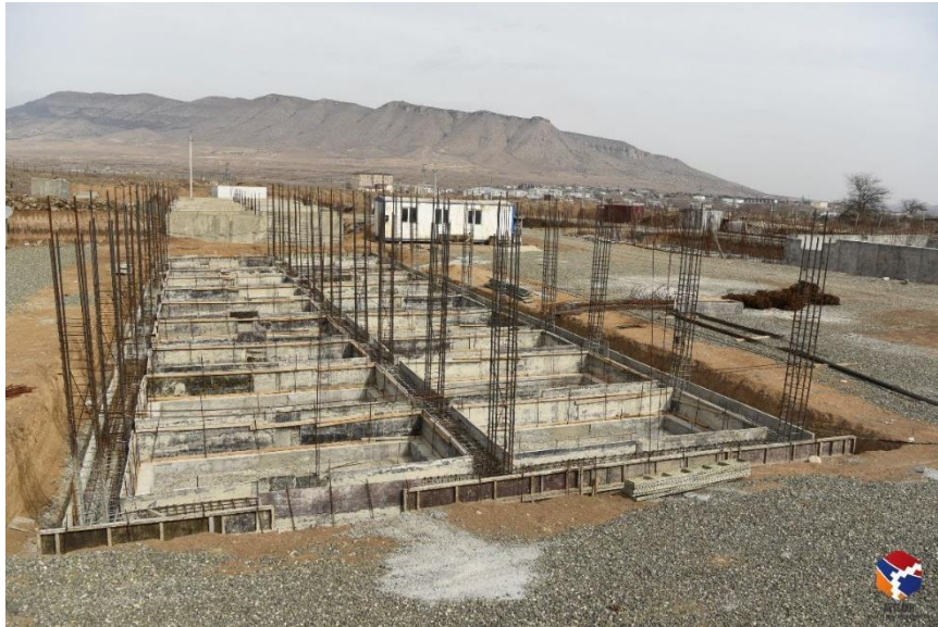
Image 22: The construction of the apartments for the displaced people are suspended
